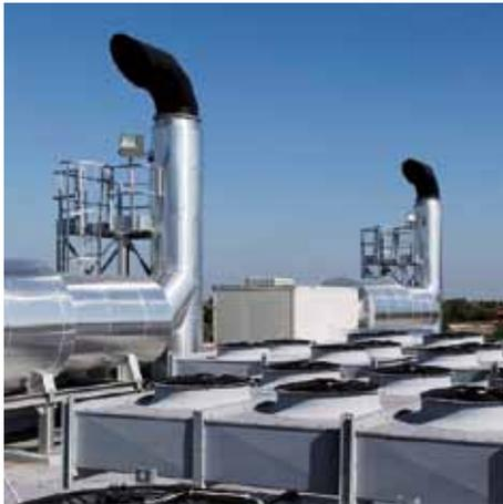
Power house at the Cereal Docks works in Camisano Vicentino in northern Italy. Cooling radiators are located on the power house roof
